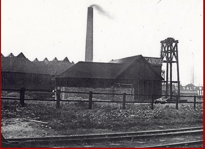
View of the Murgatroyd Works from the south-east in 1905, showing the boiler house (centre) and gantry head and shaft (right). The photograph shows what appears to be a flywheel or a winch on the eastern side of the shaft.
